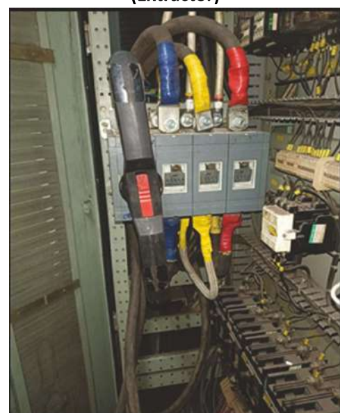
Three Way Knife Switch (Pusher)
