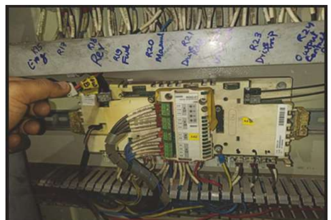
Switches and 3-way Terminal Blocks (TBs) to select between main and backup drives.
