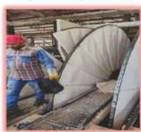
Normal Routine Segment Replacement
